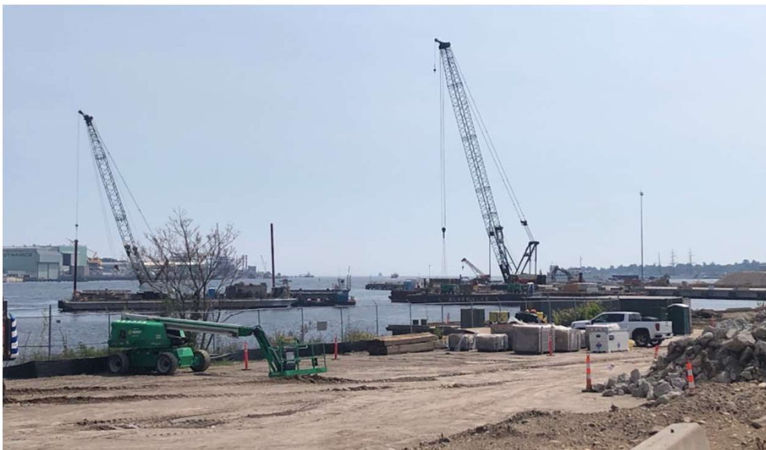
Onshore work has commenced on the New London, CT State Pier to support construction of Eversource-Ørsted offshore wind projects
